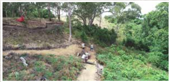
Photo: Bunya Mountain Murri Rangers Refurbishing Walking Tracks at Fishers Lookout
