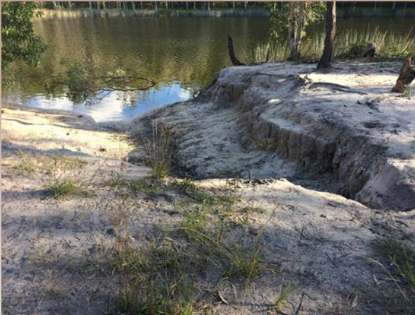
Erosion on lagoon bank
